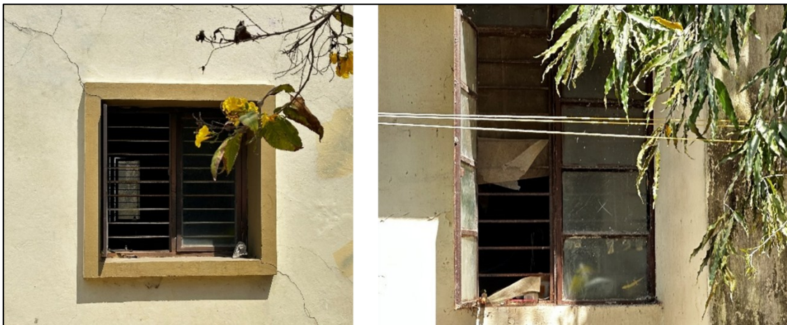
Figure 16 Existing Condition of Windows in Hostels
