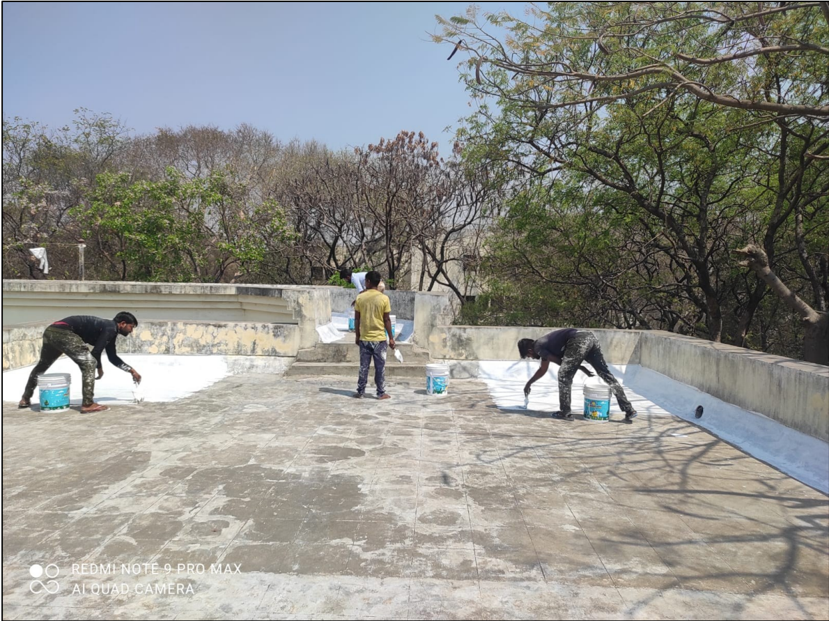
Figure 9 Cool Roof Painting During Progression
