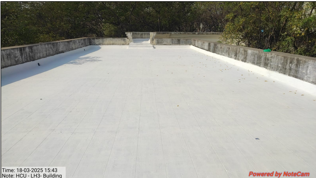
Figure 10 Cool Roof Painting After Completion
